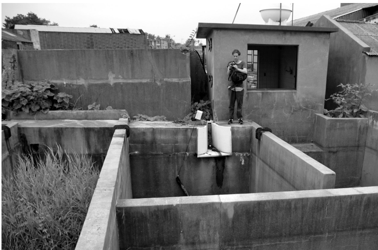
Tyler shows me around an abandoned water treatment plant.
